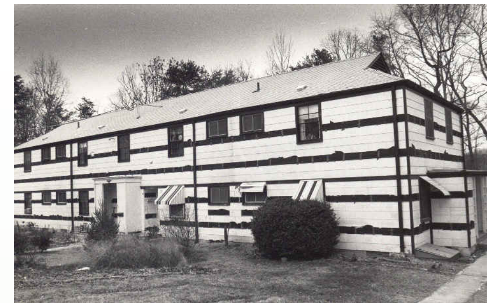
Greenbelt Homes, Incorporated begins a major rehabilitation of the cooperative's frame homes. Vinyl siding was installed to replace the original shingles. Greenbelt News Review, photograph by J. Henson
